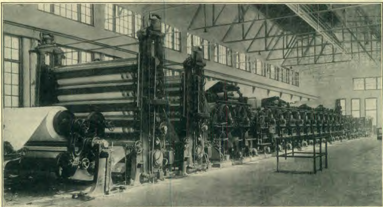
The Dry End of a Mammoth Paper Machine. It Operates on the Principle of a Laundry Mangle
