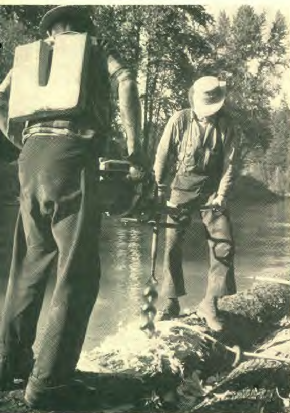
Huge drill bores holes for chains through "boomsticks" that form frame of raft. Cross pieces ("swifsters") hold raft together on trip to mill.
