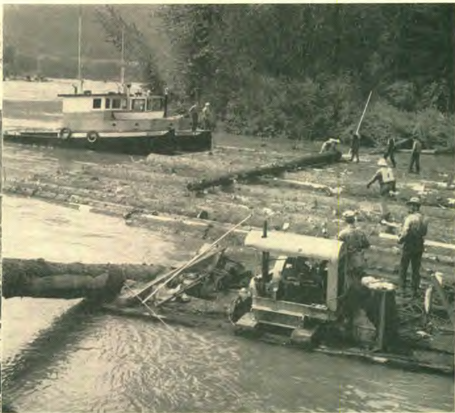
Huge drill bores holes for chains through "boomsticks" that form frame of raft. Cross pieces ("swifsters") hold raft together on trip to mill.
