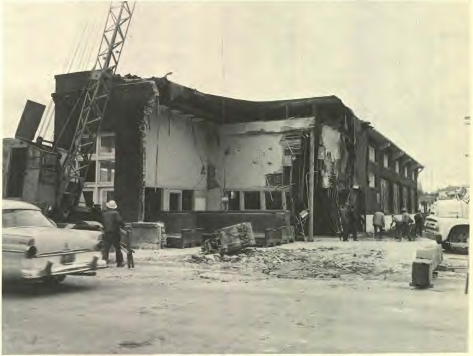
The front of the depot showed that clean-up operations had almost been completed.
