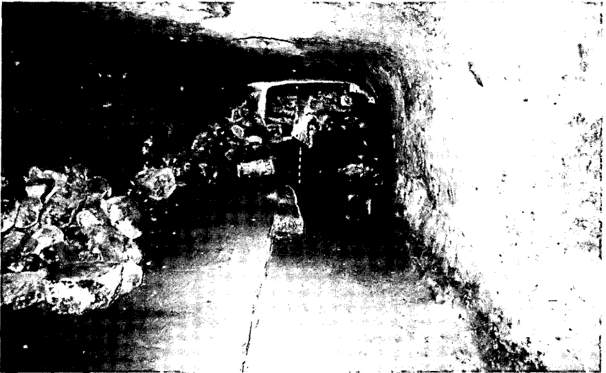
B. Square G.4. View to south. Looking down long axis of cistern past Loci G.4:5, 6, 8. Photo: Paul H. Denton.
