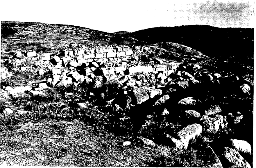
A. Site 138. View to northwest. Complex of walls within which were patches of mosaic, an apsidal wall, and two tomb entrances. Photo: Paul H. Denton and Andrew Kramer.
