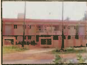
South Tamil Section Office Building
