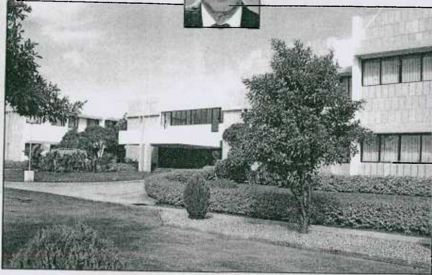
Southern Asia Division Administrative Complex of SDA, Hosur.
