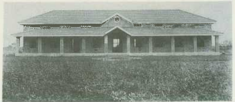
Boys dormitory, Lasalgaon, Maharashtra.
