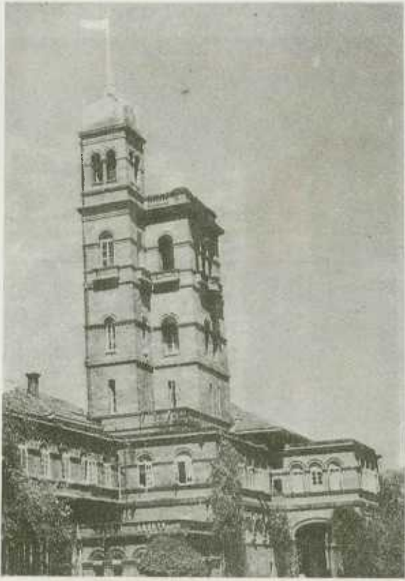
University of Pune- Administration building
