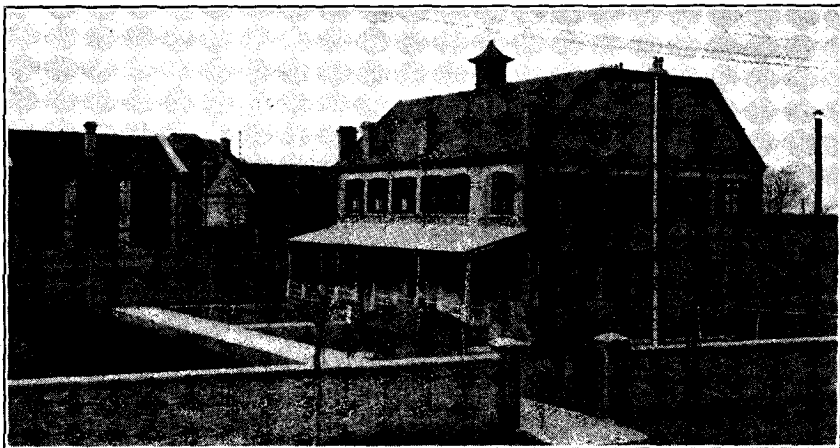
PUBLISHING HOUSE IN SHANGHAI, CHINA
