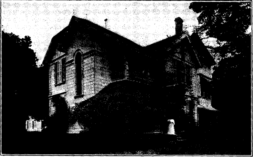
"ELMSHAVEN," HOME OF MRS. E. G. WHITE, NEAR ST. HELENA, CALIFORNIA
