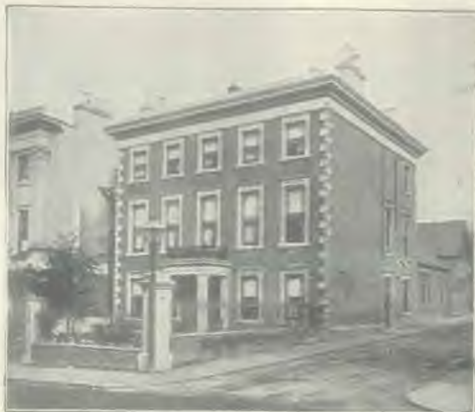
Belfast Sanitarium, Ireland.
