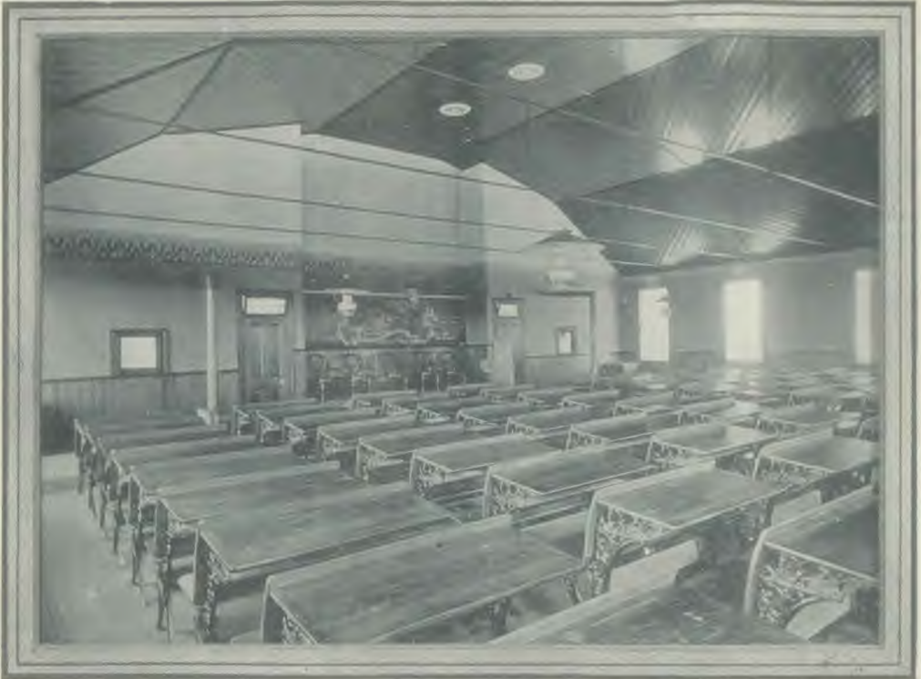
THE ASSEMBLY ROOM OF THE CENTRAL SCHOOL BUILDING.
