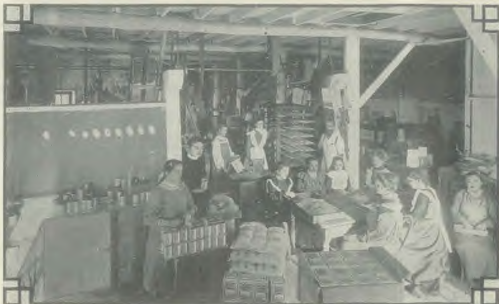
Packing Room of Sanitarium Health Food Factory.
