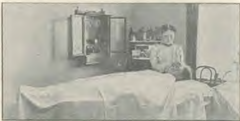
Electrical Treatment at Sydney Sanitarium.
