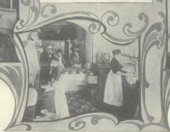
Part View of Kitchen.
