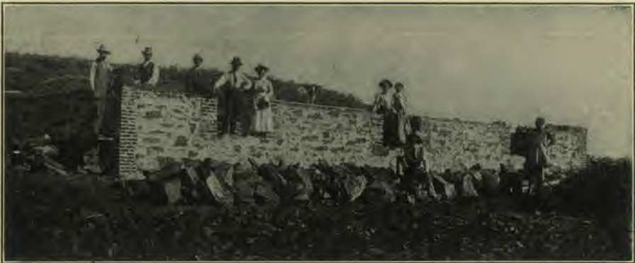
BUILDING THE NEW ASMARA MISSION HOUSE, ABYSSINIAN STATION
