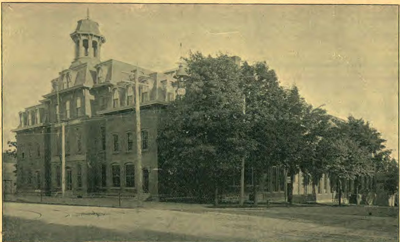
REVIEW AND HERALD PUBLISHING ASSOCIATION, BATTLE CREEK, MICH. Taken before the fire which destroyed this building, Dec. 30, 1902.
