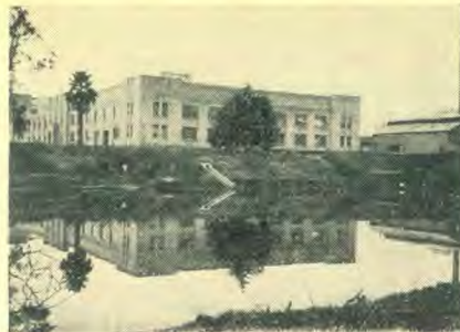
Sanitarium Health Food Company. The Old Factory Building From the South
