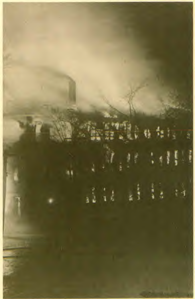
On December 30, 1902, a fire of unknown origin broke out in the Battle Creek plant. The building and its contents were a total loss.
