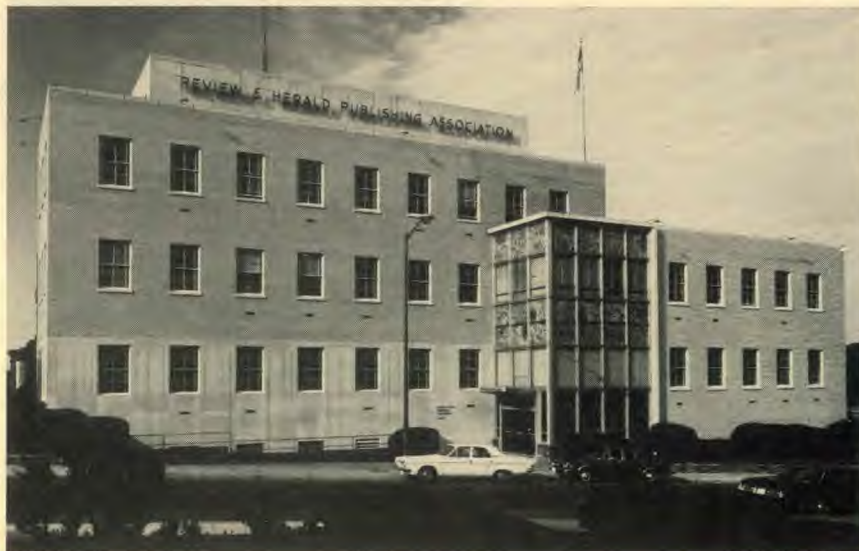
Left: Many additions have been made to the Review and Herald building in Washington, D.C., through the years, including the four-story steel, concrete, and brick addition that gave the building its present facade in 1956. The most recent addition, on the back end of the building, was completed in 1973. Above: Charles Boyd, a Review employee for 33 years, works at the casing-in machine in the bindery on the new additional ground floor.
