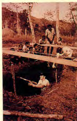
PUC students build a suspension bridge in a remote Indonesian village.
