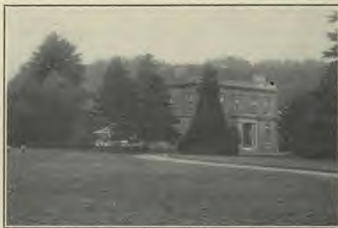
FIRST BUILDING OF THE STANBOROUGH PARK MISSIONARY COLLEGE, WATFORD, ENGLAND New buildings in process of erection.
