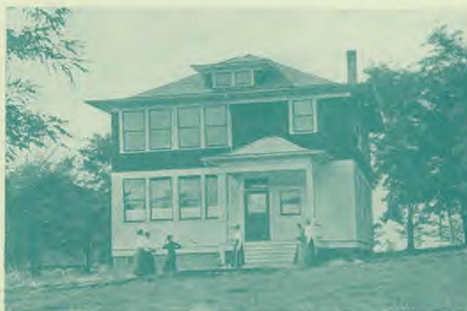
THE NORMAL BUILDING
