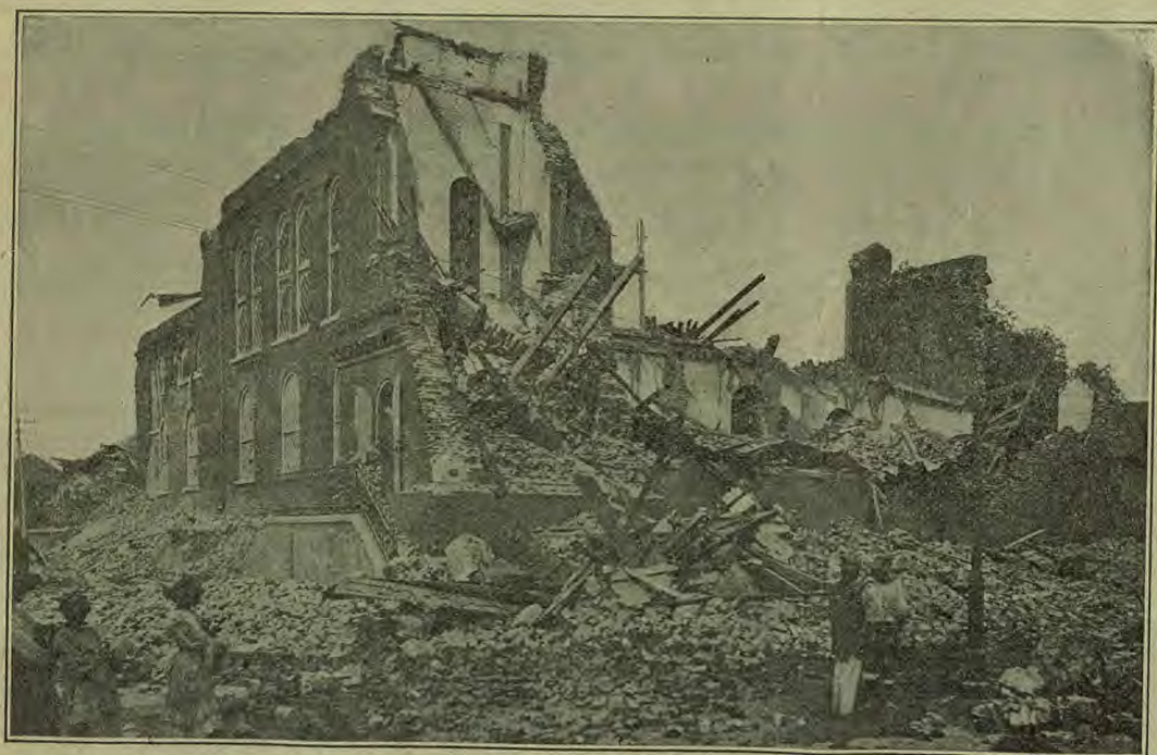
Trinity Roman Catholic Church, Kingston, Jamaica, after Earthquake of January 14, 1907.
