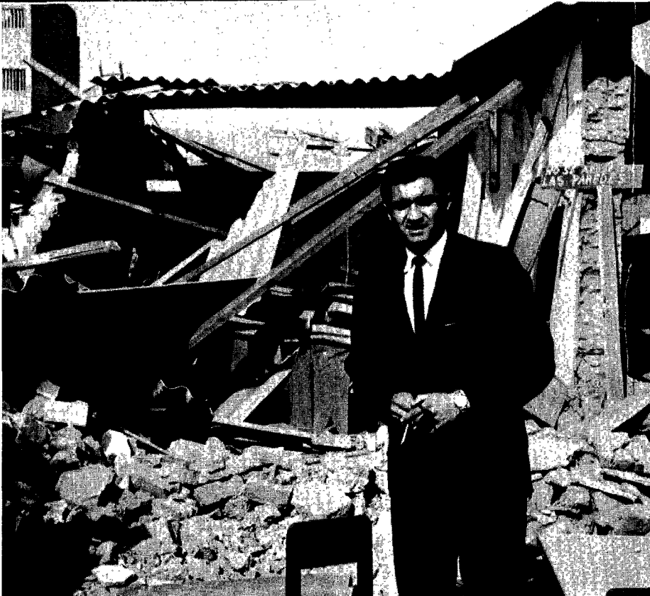
Gillermo Bonilla, SAWS public relations worker, stands in front of the rubble of the church and school in Chimbote. The hand-lettered sign says, "Don't lean on the walls."
