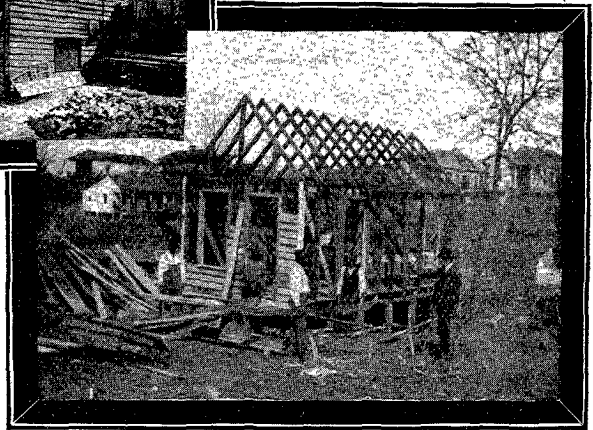
No. 5. Janitor's Cabin in Process of Building.
