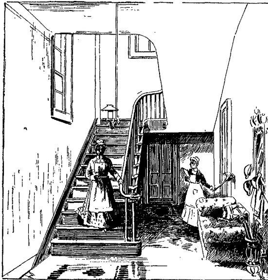
Main Hall and Stairway, Sanitarium.
