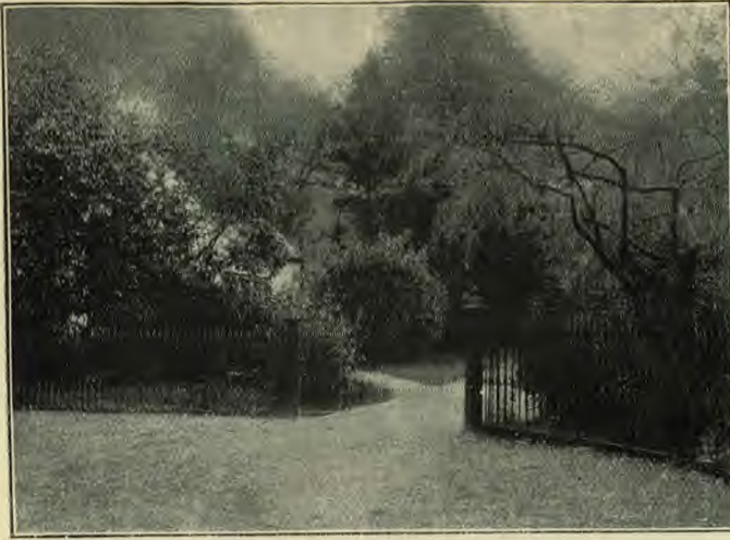
ROSTREVOR HYDRO, ENTRANCE WITH LODGE.
