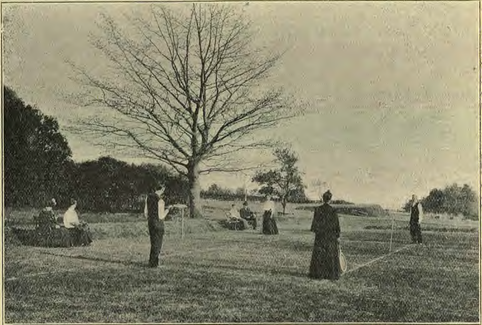
IN THE GROUNDS OF THE HYDRO.
