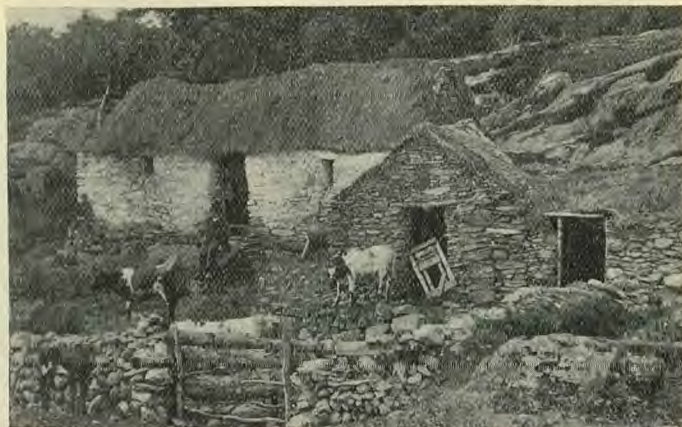
Old cottages to be displaced by those being built by Boards of Guardians.
