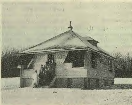
Some authorities favour a collection of cottages in preference to a single large building for the treatment of consumptives. This cottage was designed by Samuel G. Dixon, Health Commissioner for the State of New York, and we reproduce it here by the kind permission of the "Journal of the Outdoor Life." The cottage is built of wood, is 27 x 24 feet, and accommodates two persons in each of the four equal rooms into which it is divided. There is a central entry 4 ft. 8 in. in width, enlarged in the centre by cutting off the corners of the rooms, for heating and lavatory purposes. Dampness is provided against.
