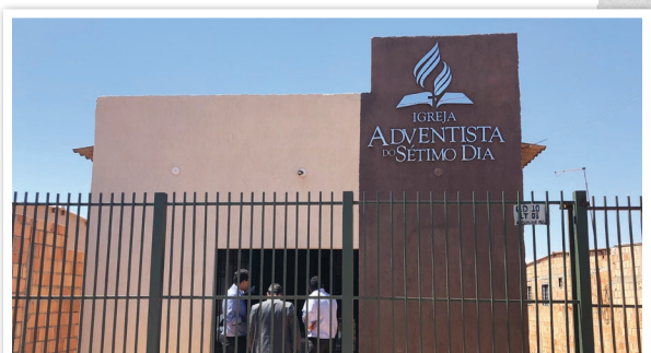
The new Adventist group in Alpha Ville bought this building from another church that closed. The new group put a new front on the church building, and now services take place regularly here.
