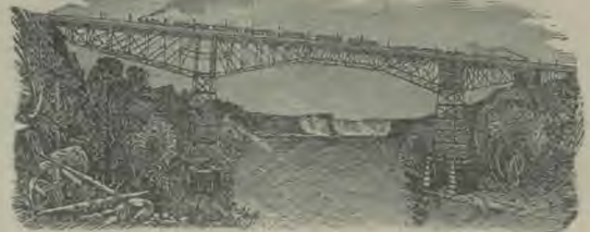
MICHIGAN CENTRAL NEW CANTILEVER BRIDGE, NIAGARA FALLS.
