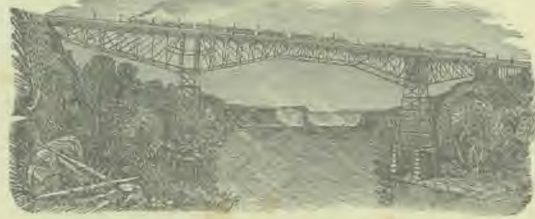
MICHIGAN CENTRAL NEW CANTILEVER BRIDGE, NIAGARA FALLS.
