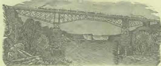
MICHIGAN CENTRAL NEW CANTILEVER BRIDGE, NIAGARA FALLS.
