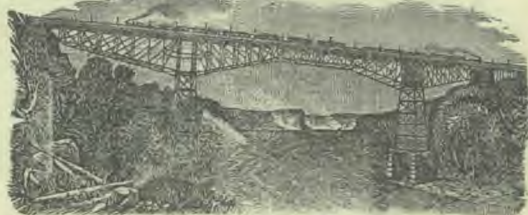
MICHIGAN CENTRAL NEW CANTILEVER BRIDGE, NIAGARA FALLS.
