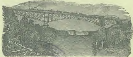
MICHIGAN CENTRAL NEW CANTILEVER BRIDGE, NIAGARA FALLS.
