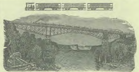
MICHIGAN CENTRAL NEW CANTILEVER BRIDGE, NIAGARA FALLS.
