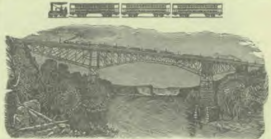
MICHIGAN CENTRAL NEW CANTILEVER BRIDGE, NIAGARA FALLS.
