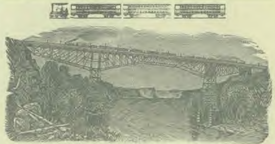
MICHIGAN CENTRAL NEW CANTILEVER BRIDGE, NIAGARA FALLS.
