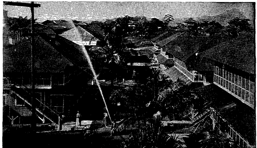
Buildings of the West Caribbean Training School
