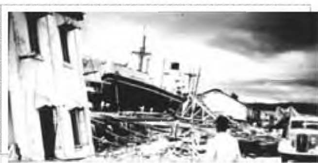
Suva Harbour after the cyclone
