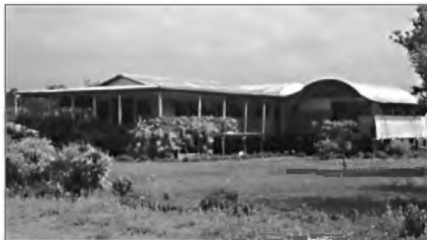
The principal's house built by Thrift out of Quonset huts
