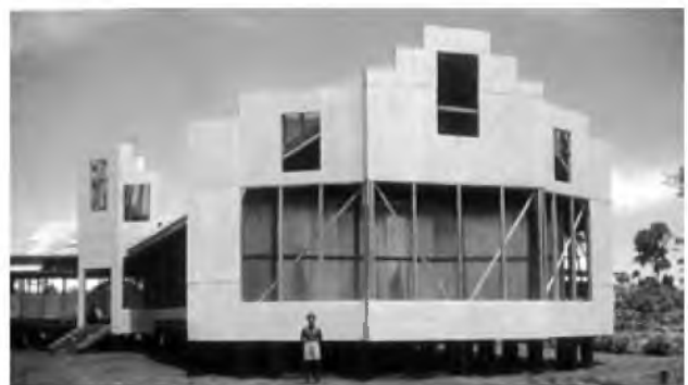
The chapel being built.
