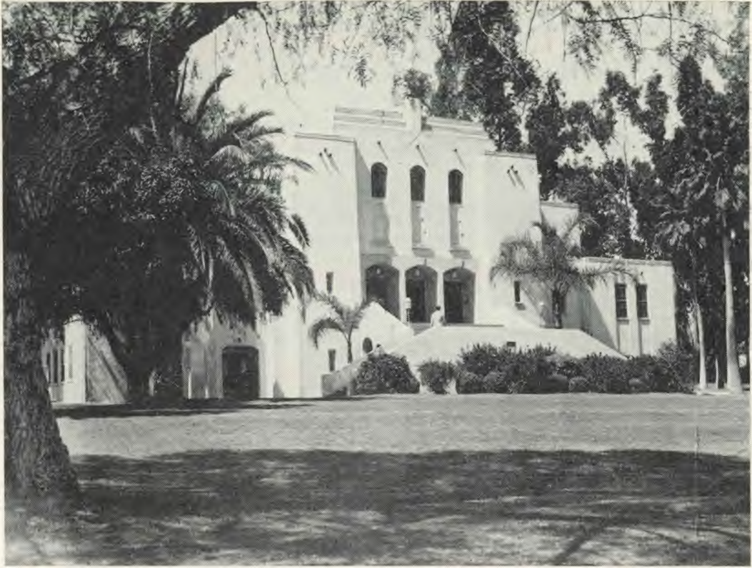
Hole Memorial Auditorium
