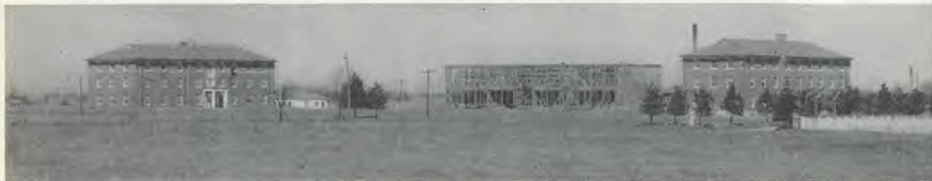
Sunnydale Academy, Centralia, Missouri. Administration Building Under Construction
