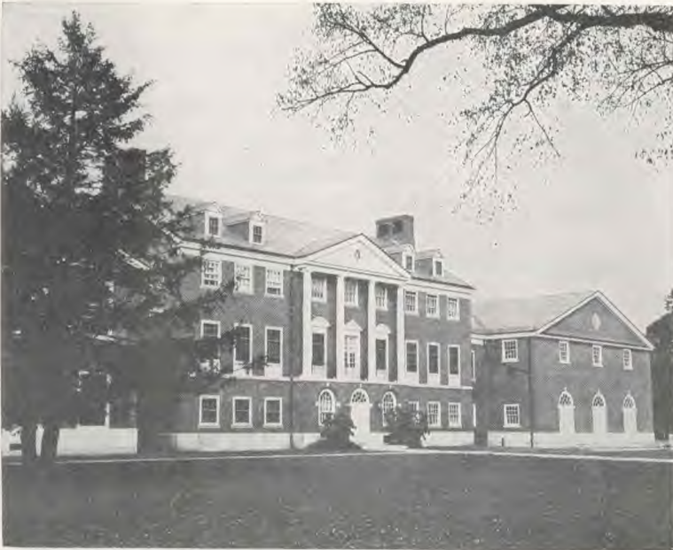
Haskell Hall—Administration Building
