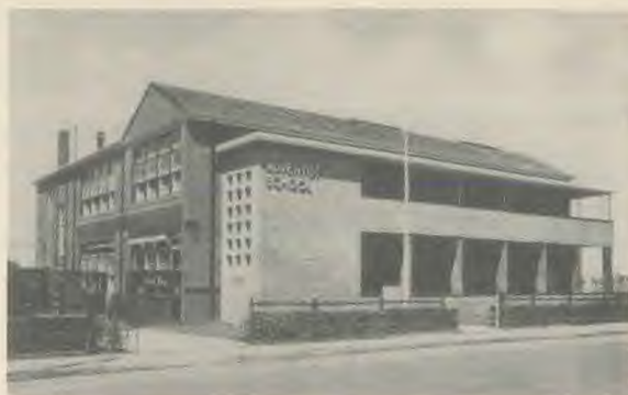
The Hawthorn School, Melbourne, Victoria
