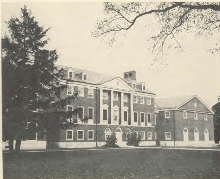
Haskell Hall—Administration Building
