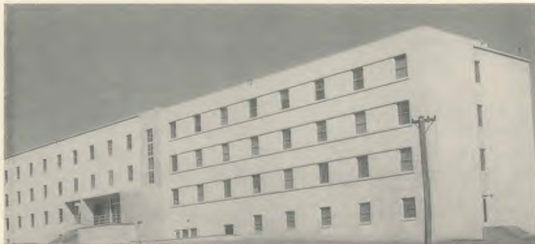
Ellen Harmon Hall—Women's Residence (Completed 1954) Latest in a series of fine new buildings added to the campus.
