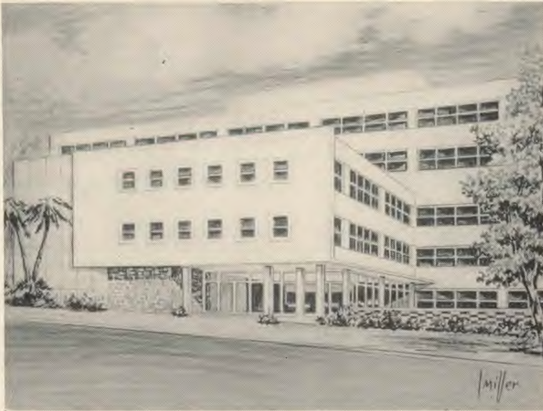
New White Memorial Hospital, Los Angeles Campus
