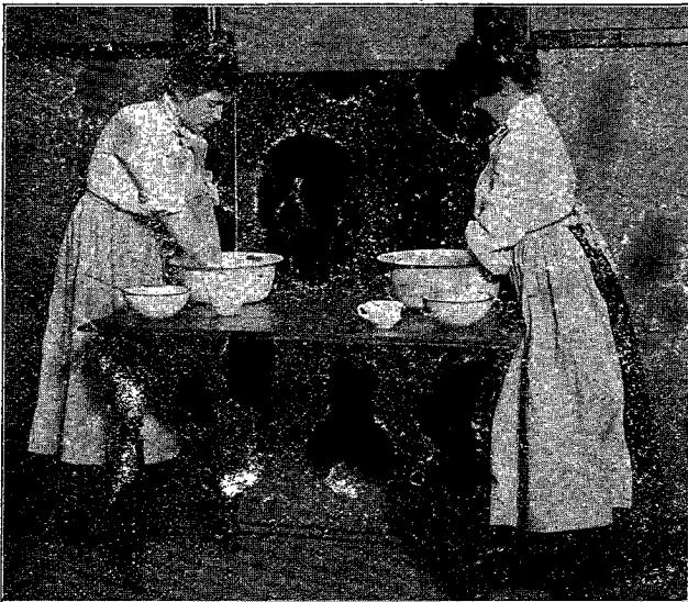
CORRECT AND INCORRECT POSITIONS.
