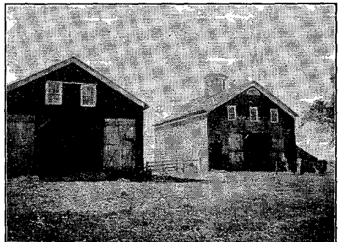
BARN ON THE FARM.
