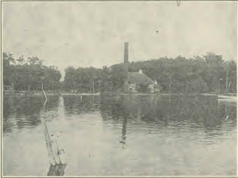
PUMPING STATION — LAKE GOGUAC
