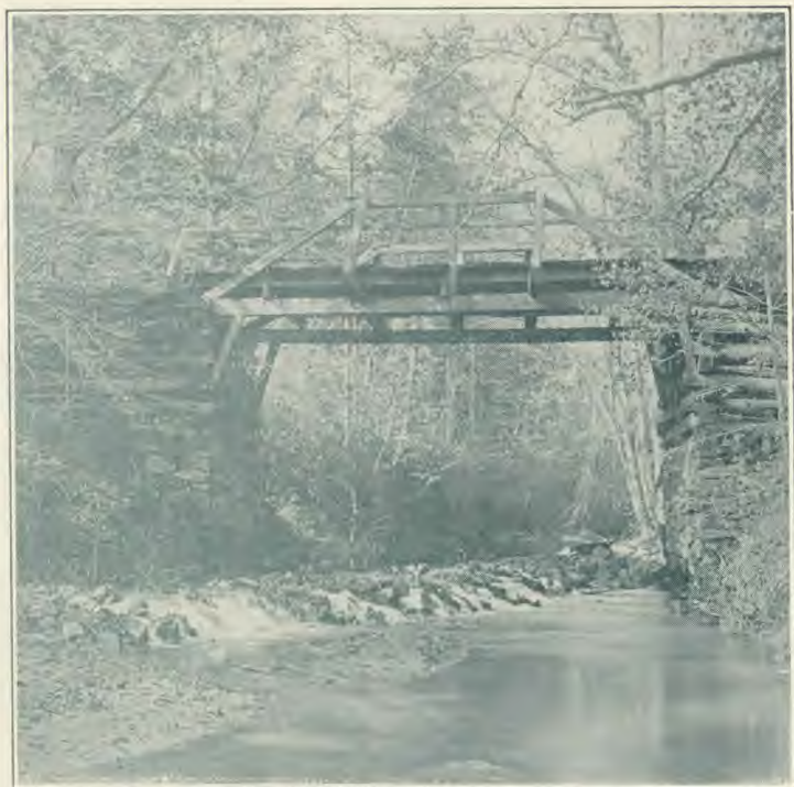
SLIGO BRIDGE, TAKOMA PARK, D. C.
