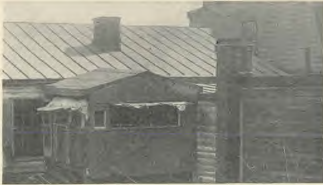
Outdoor sleeping-room. This was built by the patient on his own roof; cost, about six dollars
